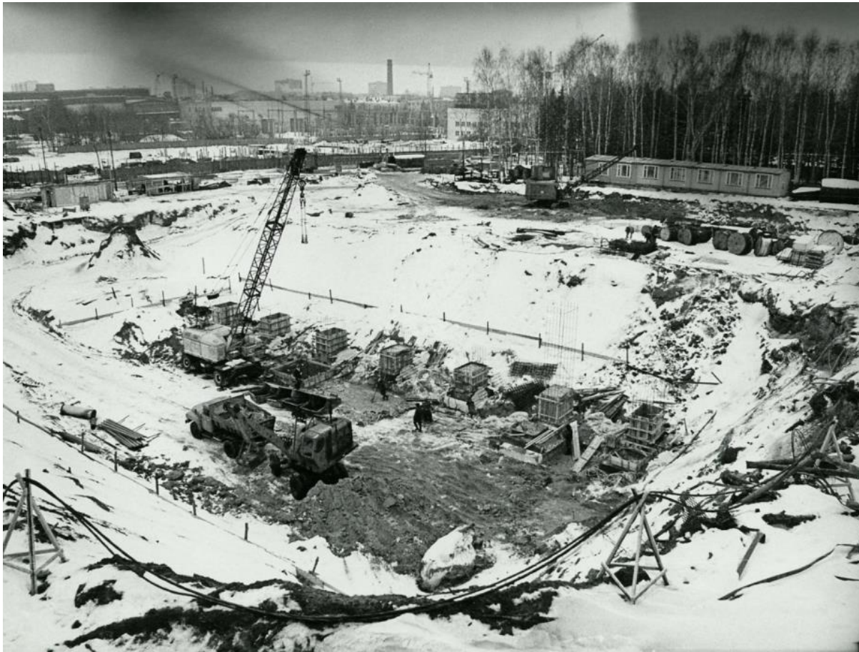
The Kurchatov synchrotron foundation laying (December 1985, Soviet Union)
